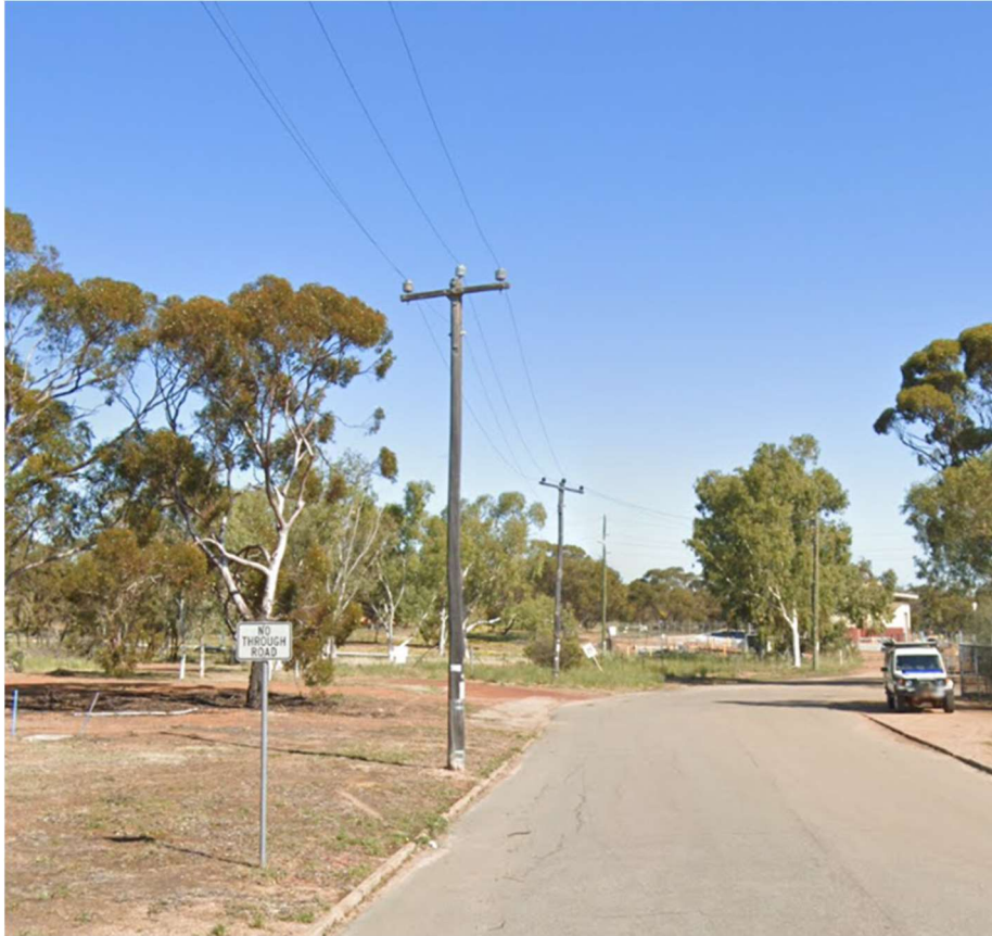
Figure 5: WP Overhead Assets on Mitchell St
